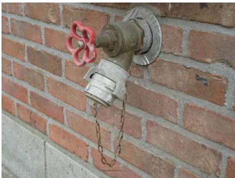
Figure 19 : Hydrant mural ou raccord DSP Ø45mm seul
